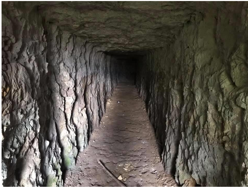
Tunnel below the Pagoda for communications.
